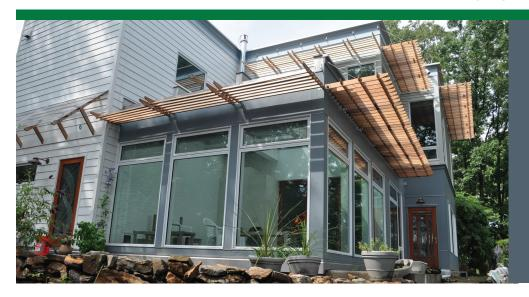
Nearly every room and closet in the home receives natural light through triple-pane low-emissivity windows or insulated solar tubes. Extra attention to air sealing helped the home achieve a very low air leakage rate of 0.45 ACH 50.
