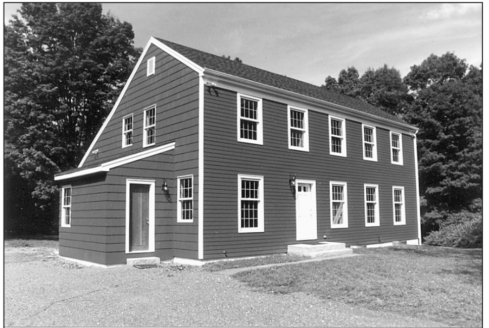
Green building is compatible with a variety of housing styles.
