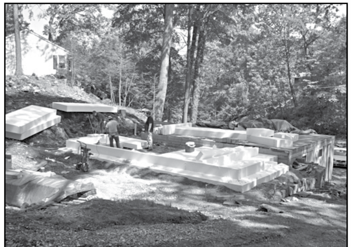
Figure 13. Shallow frost-protected foundation during assembly. Photo courtesy Mike Trolle.
