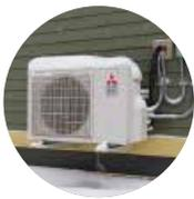
**PACKS A PUNCH** This small air-source heat pump warms the entire house with heat pulled from the winter air. It is rated for one
