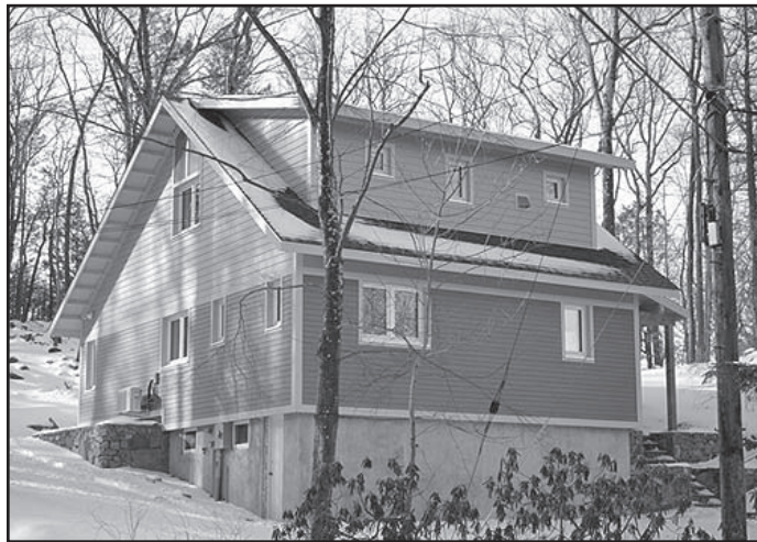
Figure 3. Exterior shot of the Trolle Residence. Trolle’s company, BPC Green Builders, has earned multiple Silver, Gold, and Platinum Leadership in Energy and Environmental Design (LEED)® for Homes certifications, and a National Green Building Standard™ (NGBS) Emerald certification. Regionally, BPC projects have been awarded “Best Energy Efficient & Green Home” in Connecticut for 2004 and 2006 (HOBBI Awards), “Best Green Renovation” in Connecticut for 2011 (Home Builders Association of CT), and “Best Use of Advanced Building Technology” Green Home of the Year Awards program ( Green Builder magazine). Trolle put the lessons from these projects together, resulting in the high performance of his personal residence. Photo courtesy Mike Trolle.
