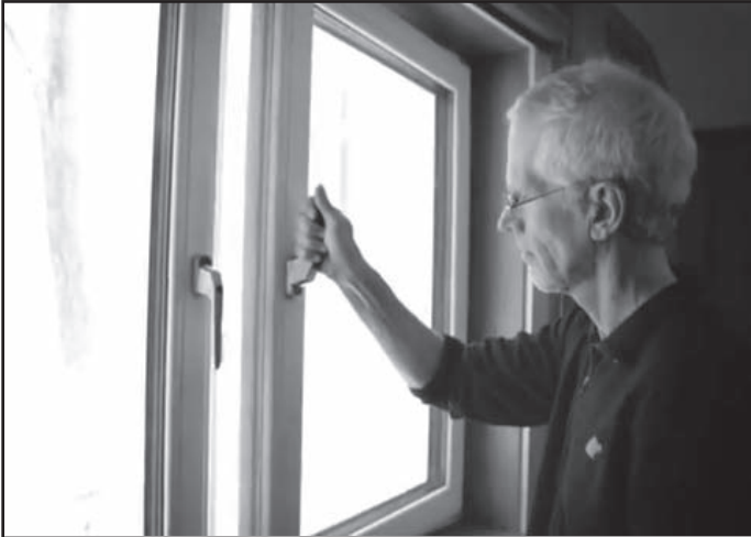
Figure 5. The Klearwall (Munster Joinery) windows selected for the project have proved exceptional, both in U-value, air sealing capabilities, and solar heat gain. Photo courtesy Mike Trolle. To view a video of the home, visit https://www.youtube.com/watch?v=qaLMY9QfNTc online.
