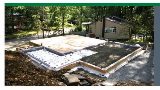
Wood subfloor covers the existing basement. A 12-inch layer of EPS rigid foam covers the remainder of the floor area, which has been prepared for pouring of the concrete slab. In the white section to the left, leftover pieces were stacked on for an additional 6 inches of foam while rock dust covers the foam in the section to the right. The 6-inch-thick perimeter slab edge insulation is covered with vapor barrier in this photo.
