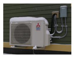
A single one-ton mini-split ductless heat pump (outdoor unit shown here) was enough to heat and cool the entire 1,650 ft² two-story home. A small duct with an inline fan helped pull conditioned air through the ceiling to upstairs bedrooms. An ERV provided fresh air ventilation and also helped to circulate conditioned air with a supply duct in the great room and return ducts in the bedrooms and bathrooms.
